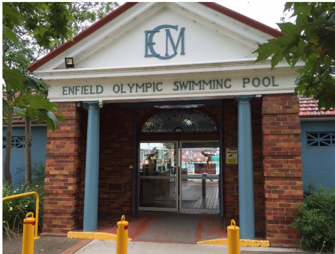
Figure 6: Entry Portico and doors with original leadlight fanlight over Bollards and handrails painted yellow are intrusive, the bases of the Doric Columns have been cemented in when constructing the access ramp.
